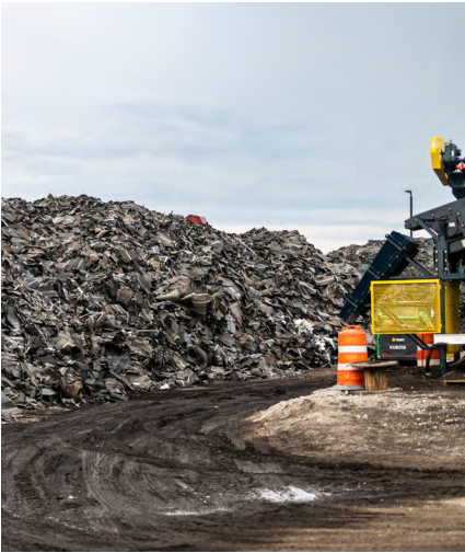
Northstar Clean Technologies secured a five-year agreement with the City of Calgary to recycle asphalt shingles from three municipal facilities.
