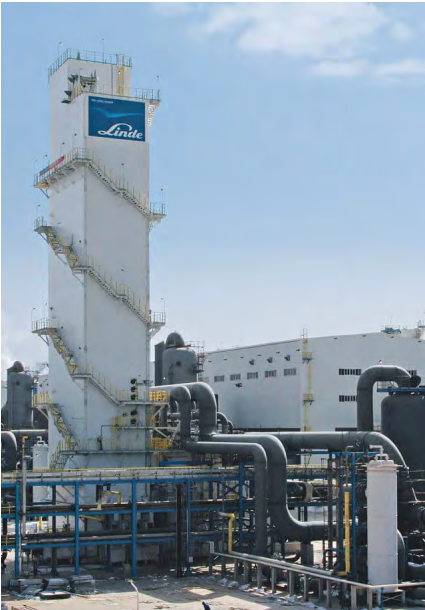
Linde's low-carbon LNG demonstration project became fully operational.
