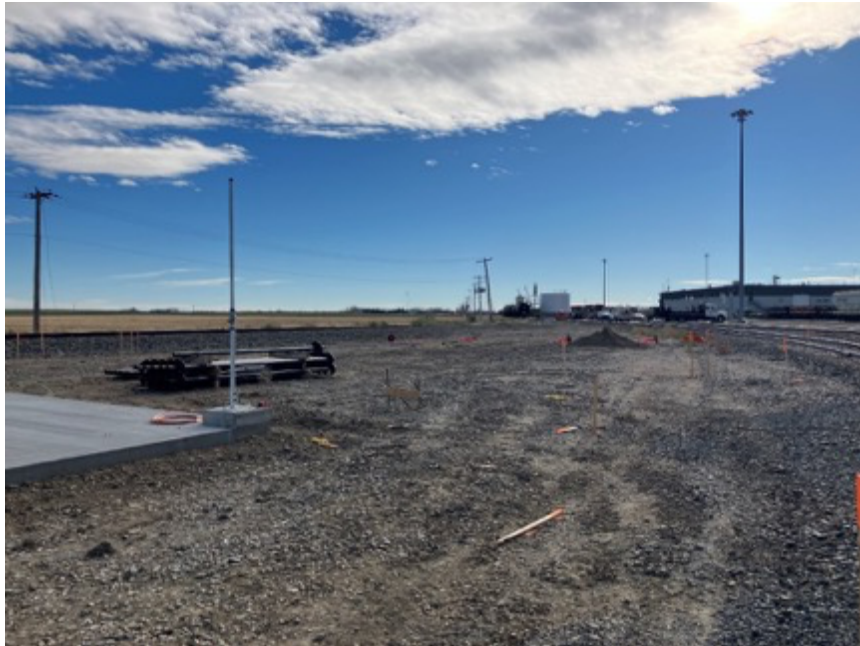
Figure 20 - Initial construction at site – grading, concrete foundation pouring.
