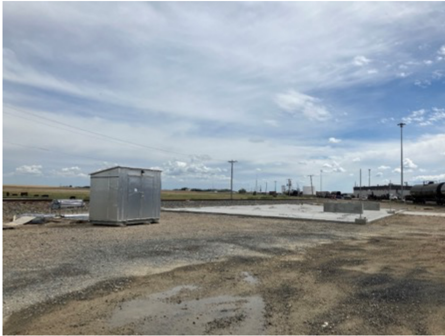
Figure 23 - Construction at Kipp Yard terminal as in August 2025
