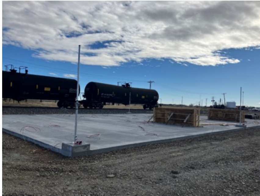
Figure 21 - Initial construction at site – concrete pouring, electrical work, lighting post installation.
