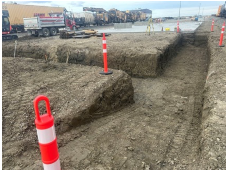
Figure 22 - Trenching for hydrogen supply line vault.
