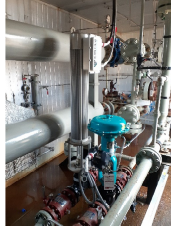
Figure 1 - Left: Dump valve actuators on a separator. Right: Kinitics prototype actuator on a gas lift valve
