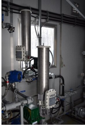
Figure 1 - Left: Dump valve actuators on a separator. Right: Kinitics prototype actuator on a gas lift valve
