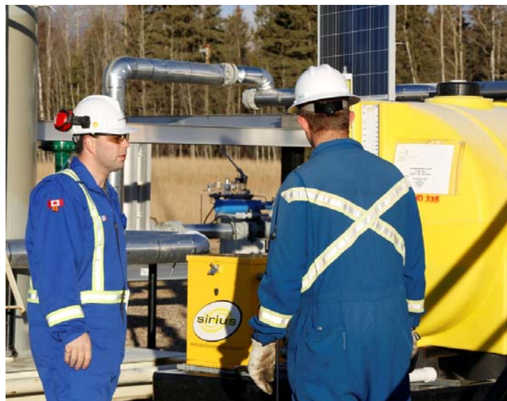
Solar Chemical Pump Installation
