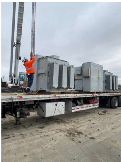
Transformer being offloaded
