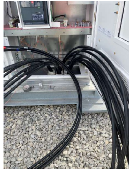
Cables pulled into inverter via conduit
