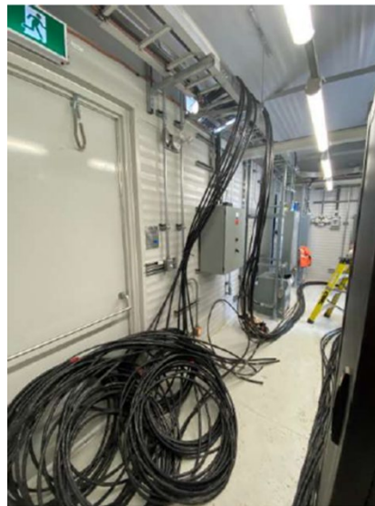
Cable pulled inside Control Enclosure
