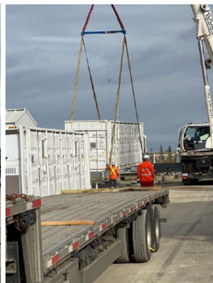
HPSU being offloaded
