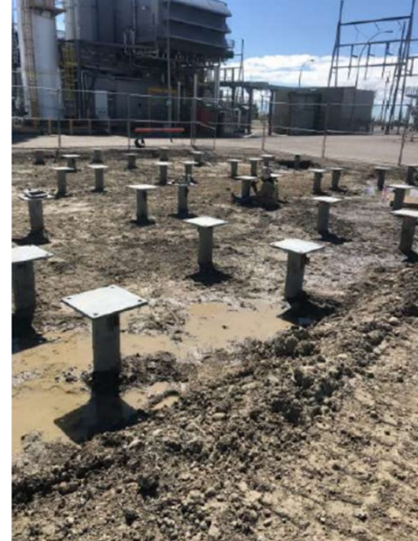
Screw piles for equipment
