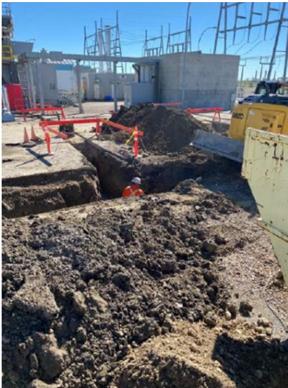
Trenches from MVSG to CRS GSU
