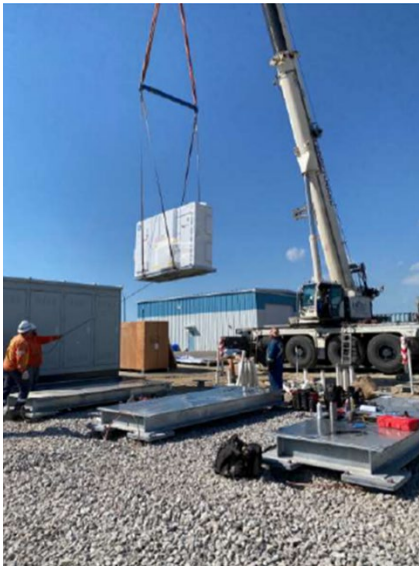
Inverter being offloaded
