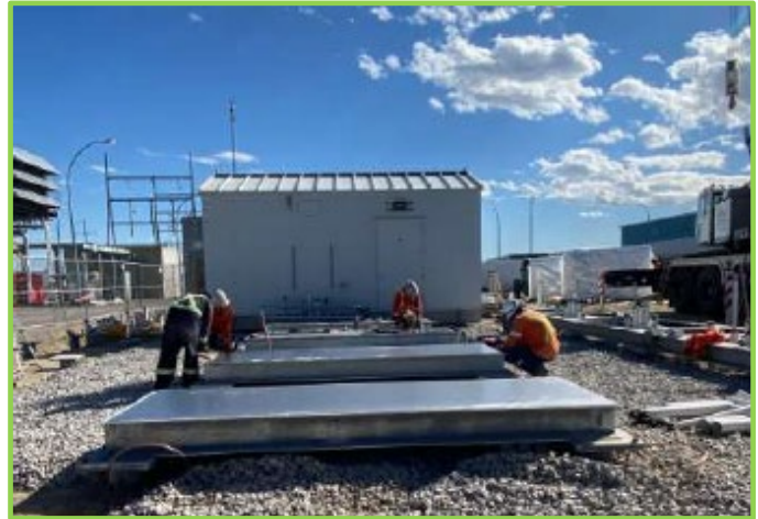
Picture of Control Enclosure Building (Centre) during construction.
