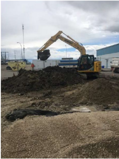
Excavation of BESS Area
