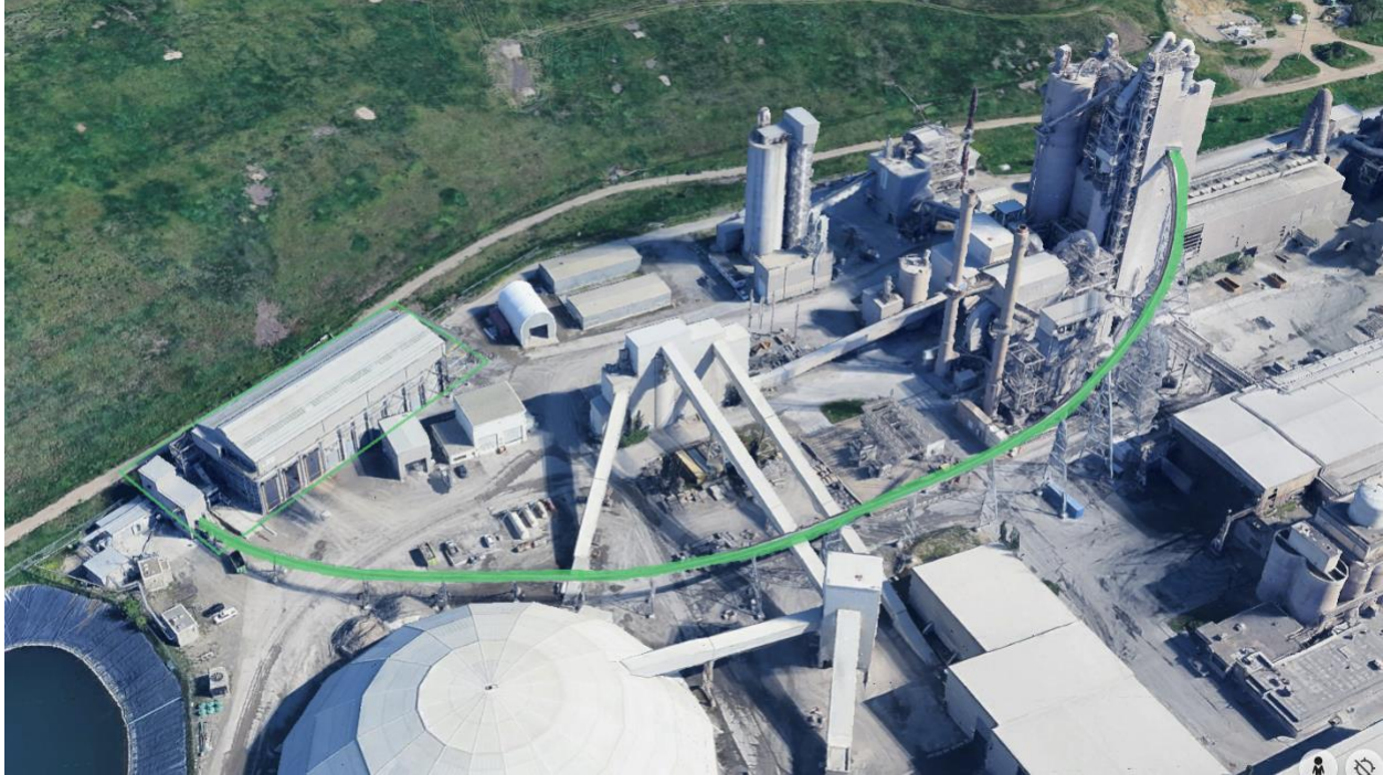
Figure 11 Overview of Project – Photo from Google Earth
