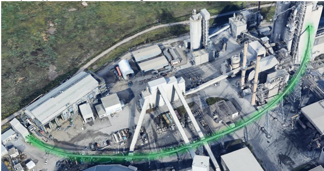
Figure 8 Tube Conveyor System - Photo from Google Earth
