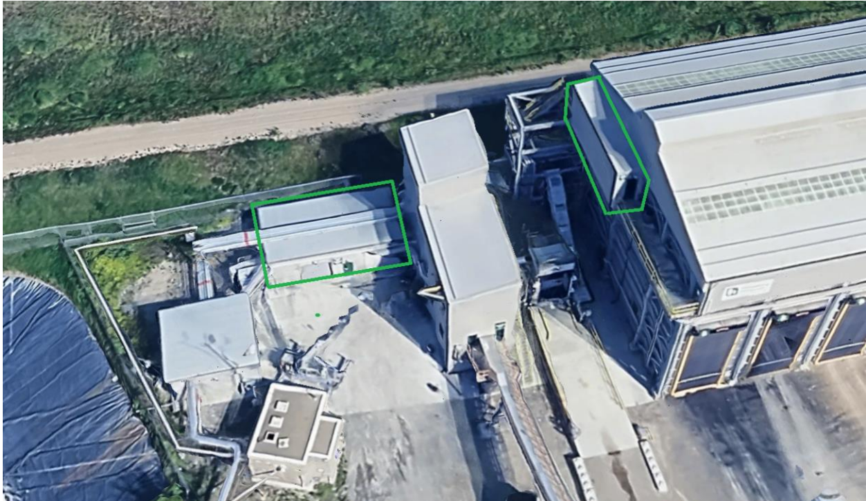
Figure 12 Electrical MCCs - Photo from Google Earth
