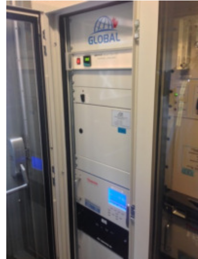
Figure 1. Global TRS CEMS instrumentation rack
