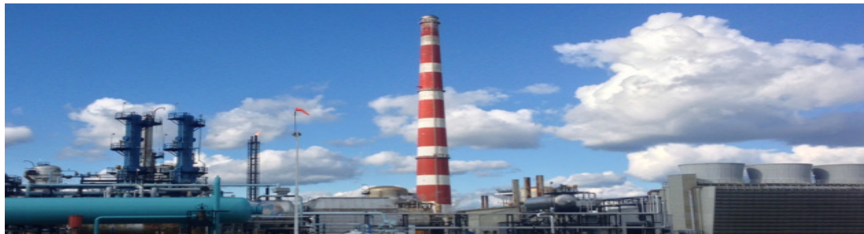
Figure 4. SemCAMS Kaybob South #3 Gas Plant, located near Fox Creek, Alberta
