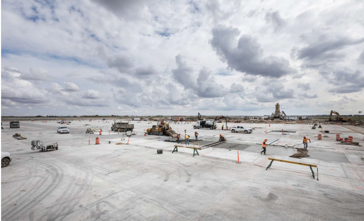
Figure 5: Work underway at Calgary International Airport using CarbonCure concrete
