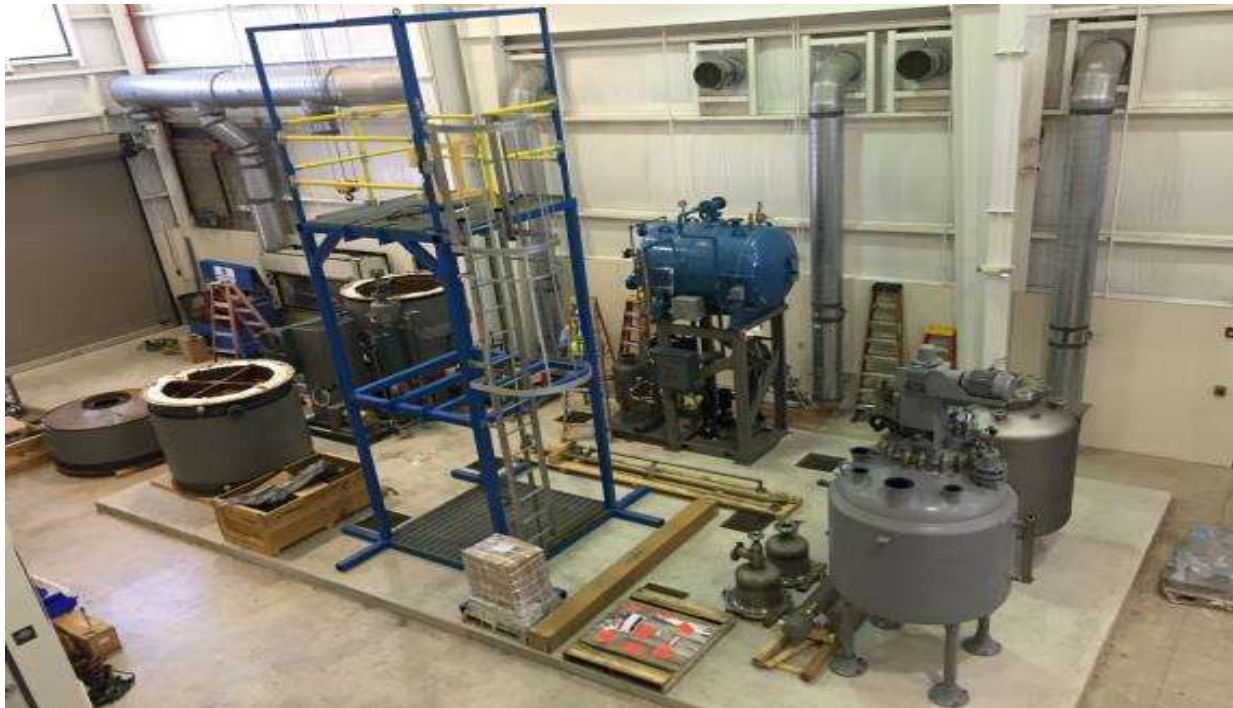
Fig. 4.2 - Beginning of SWRI SkyCycle™ Pilot Installation
