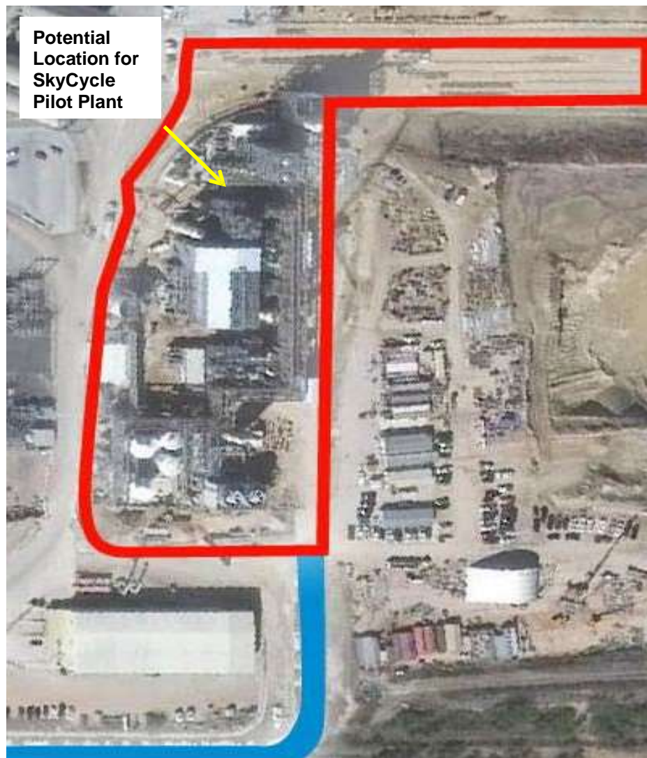
Figure 3.6 Future SkyCycle™ Commercial Pilot Plant Site at Capitol SkyMine
