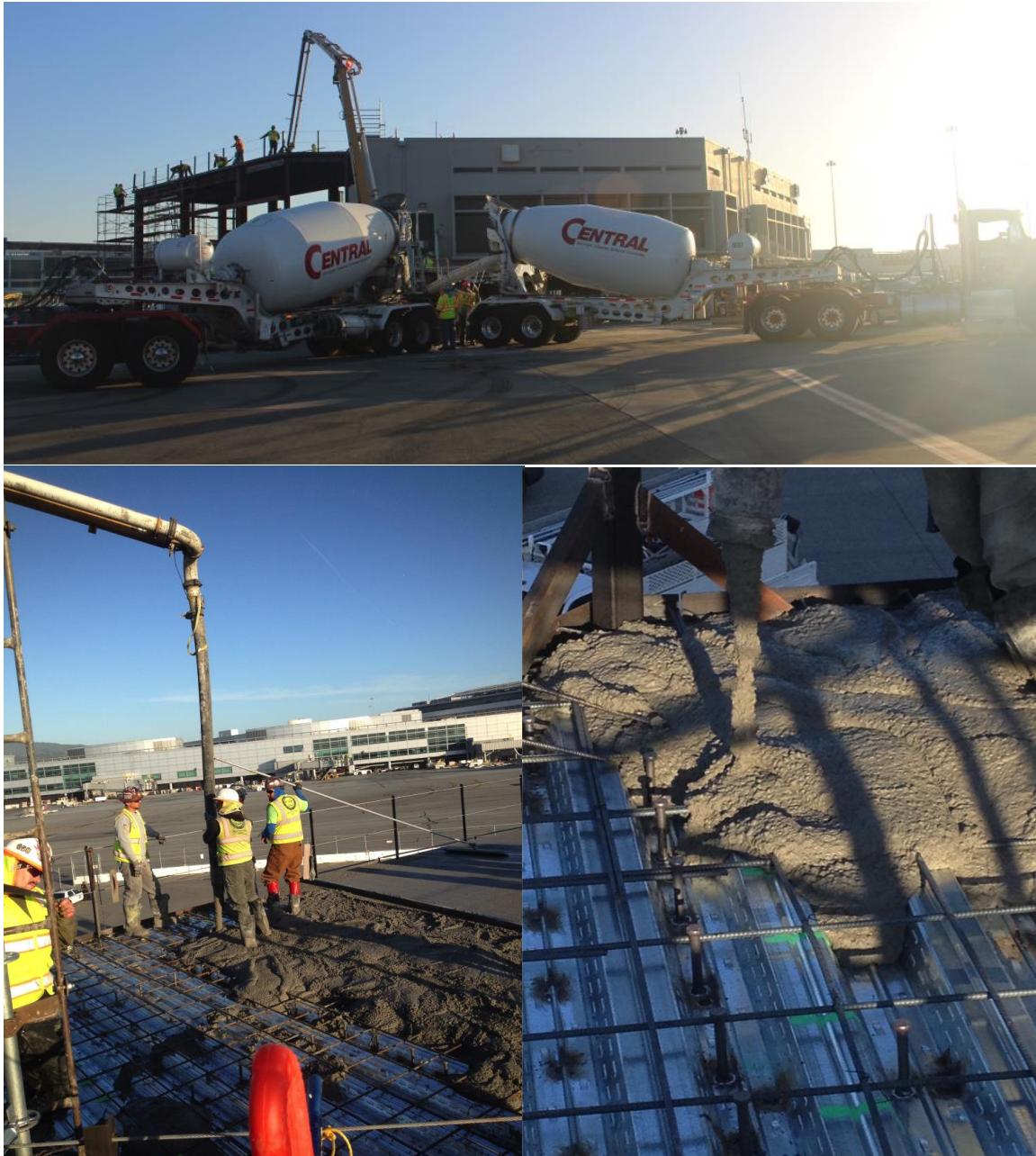
Fig. 13 Images of concrete demonstration pour by Central Concrete and using Blue Planet CarbonMix aggregate in the concrete formulation. Job summary: on the morning of May 18, 2016, Blue Planet CarbonMix lightweight aggregates (LWA) were used as a 5% LWA replacement in a mix design; materials were batched using normal methods of gravimetric feeding and discharged into ready mix trucks. The Central Concrete QA/QC lab had previously externally validated CarbonMix in Mar 2016.
