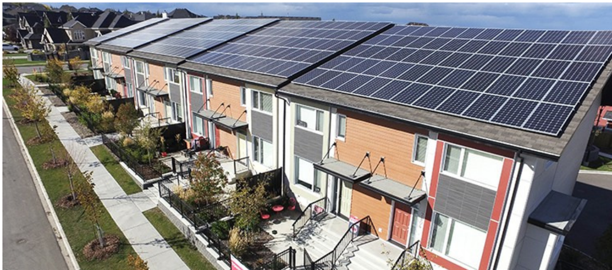
Figure 1: NetZero Energy townhomes (9-plex)
