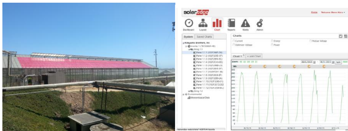
Figure 19: Final installation at KF farms of 270 Soliculture panels (left). The array provides up to 8KWac the greenhouse facility and 21 separate sections are monitored online with the inverter..
