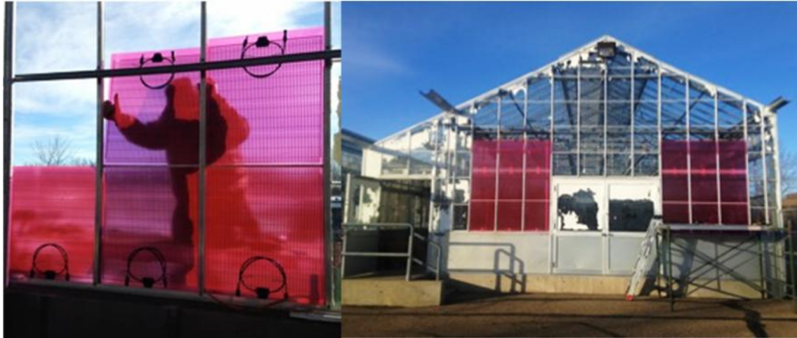
Figure 14. LUMO solar panels installed on a south-facing wall at AITF Vegreville.
