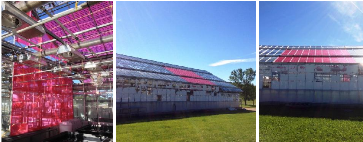
Figure 1: AITF greenhouse compartment fitted with LSC panels.
