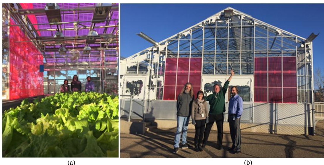
Figure 32: Greenhouse demonstration sites at AITF greenhouse in Vegreville. The combined greenhouse solar panels generates up to 1000W of power.
