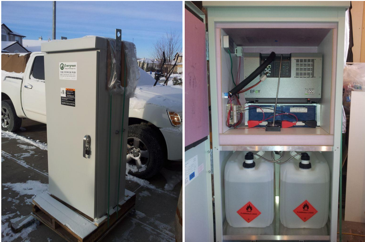
Latest Version of Power Pod (Type D) with CSA, improved exhaust, DuoCartSwitch, and (2) 28L Fuel Cartridges (61,600 Watt-hours of standby power)
