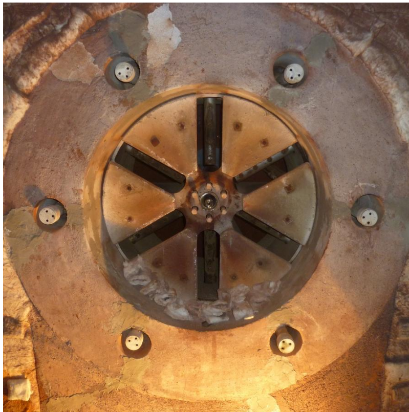
Figure 5: Coen QLN Burner with Center Praxair J-Burner (with permission from Cenovus FCCL Ltd.)
