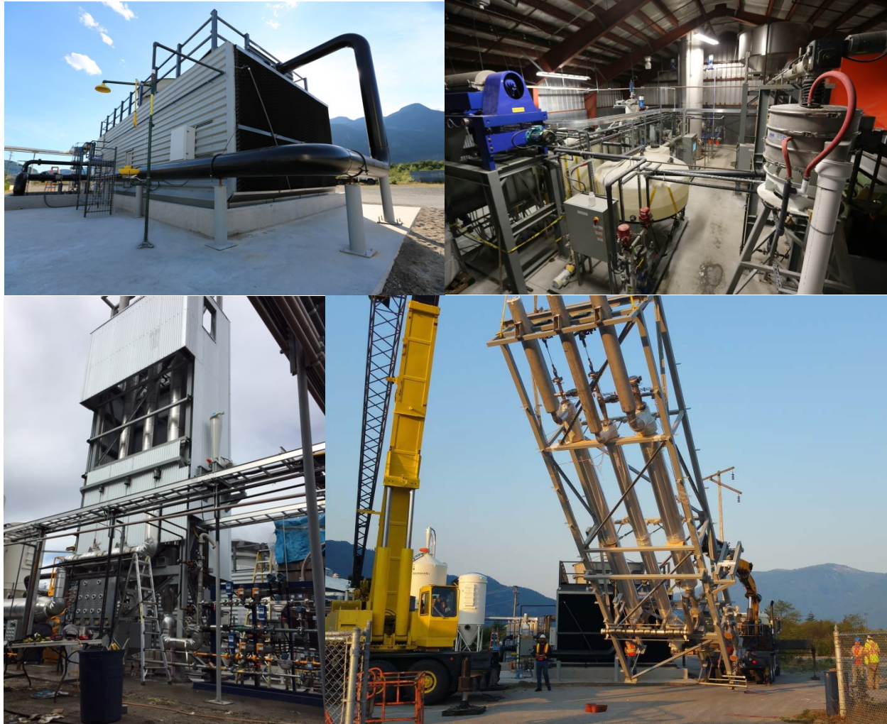
Figure 4 (clockwise from top left): Air contactor completely installed. Pellet reactor and washer/dryer area. Calciner arrival. Calciner installed with cladding in place.
