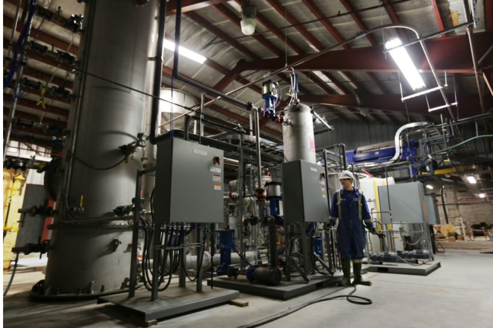
Figure 7 - Pellet reactor main vessel and seed feed system
