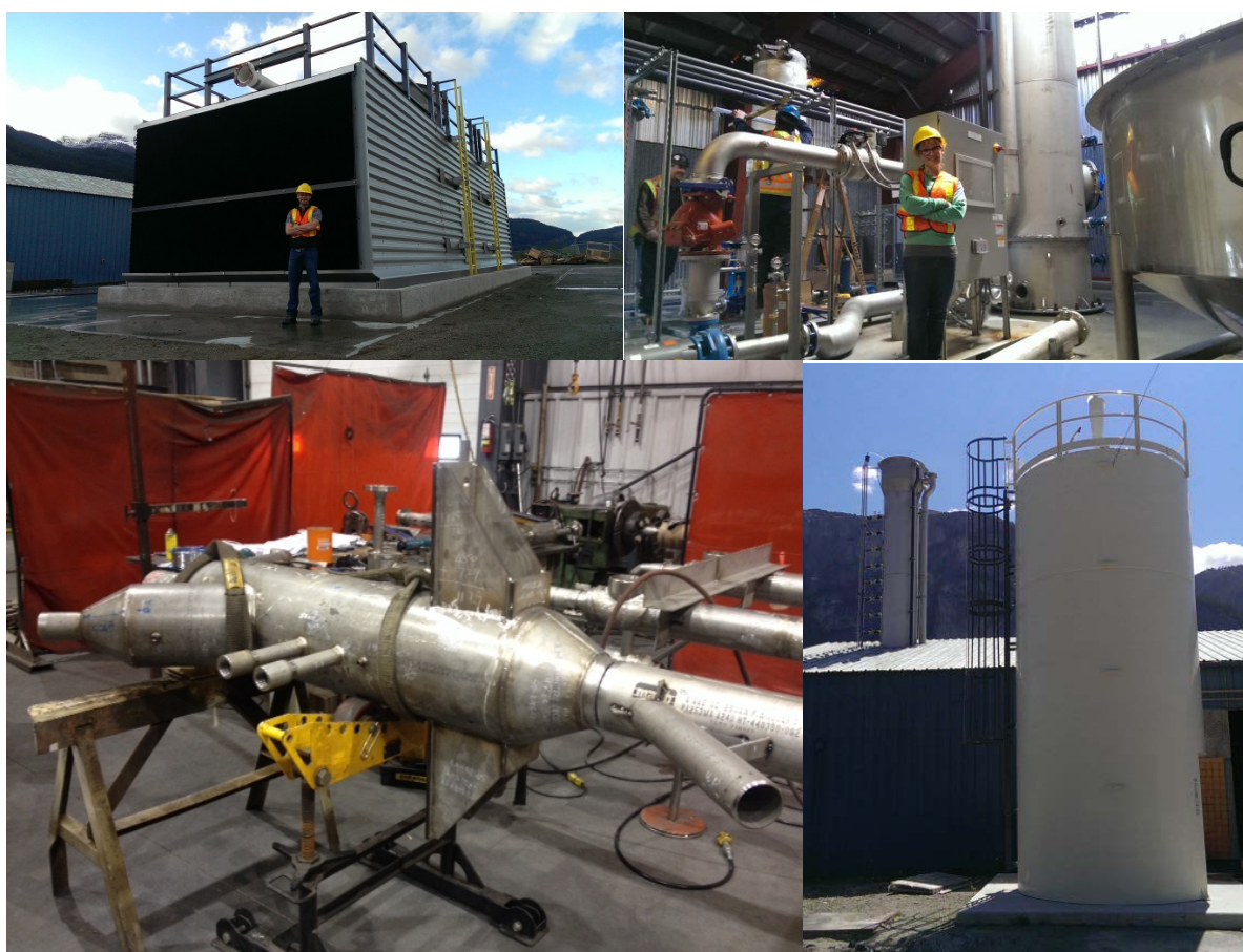
Figure 3 (clockwise from top left): Air contactor “substantial completion”. Early pellet reactor site assembly. Slaker install (there really is a slaker in there, you’ll just have to trust us). And calciner vessel fabrication progress.
